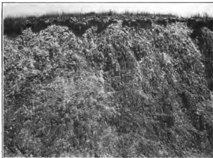
FIG. 11.—Cutting in Hudson slate decaying in place, between Shoemakersville and Hamburg, Berks Co.
